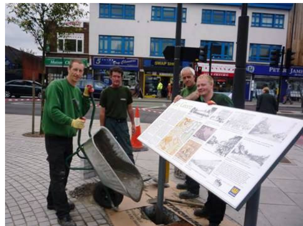
Installing the heritage panel
