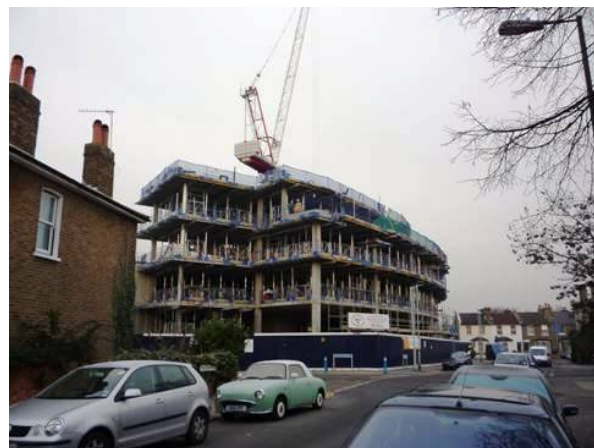
Northbrook School under construction
